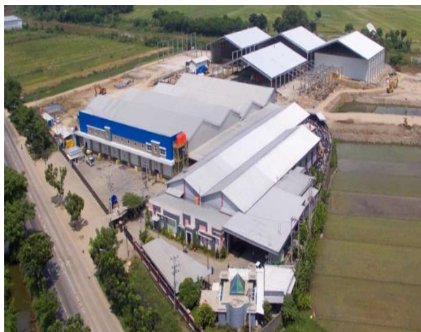
Figure 9. DPUM's facility & cold storage in Pati
